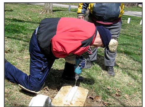
Garry Walls and Phil McClure fit a stone broken in four places. After careful measurement, holes for the copper pins are drilled and the pieces fitted, epoxied, and clamped together. After drying, the excess epoxy is shaved off and smoothed. Below Mike Beck drills at the base of another stone.
