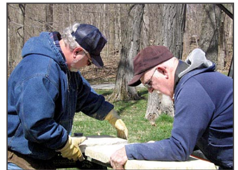
Garry Walls and Phil McClure fit a stone broken in four places. After careful measurement, holes for the copper pins are drilled and the pieces fitted, epoxied, and clamped together. After drying, the excess epoxy is shaved off and smoothed. Below Mike Beck drills at the base of another stone.
